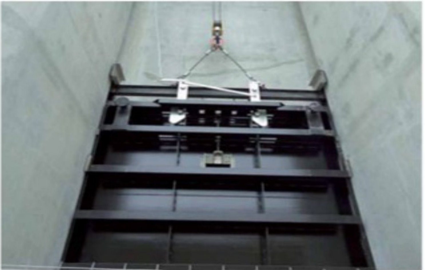
Figure Three: General Arrangement for stop logs/gates.
