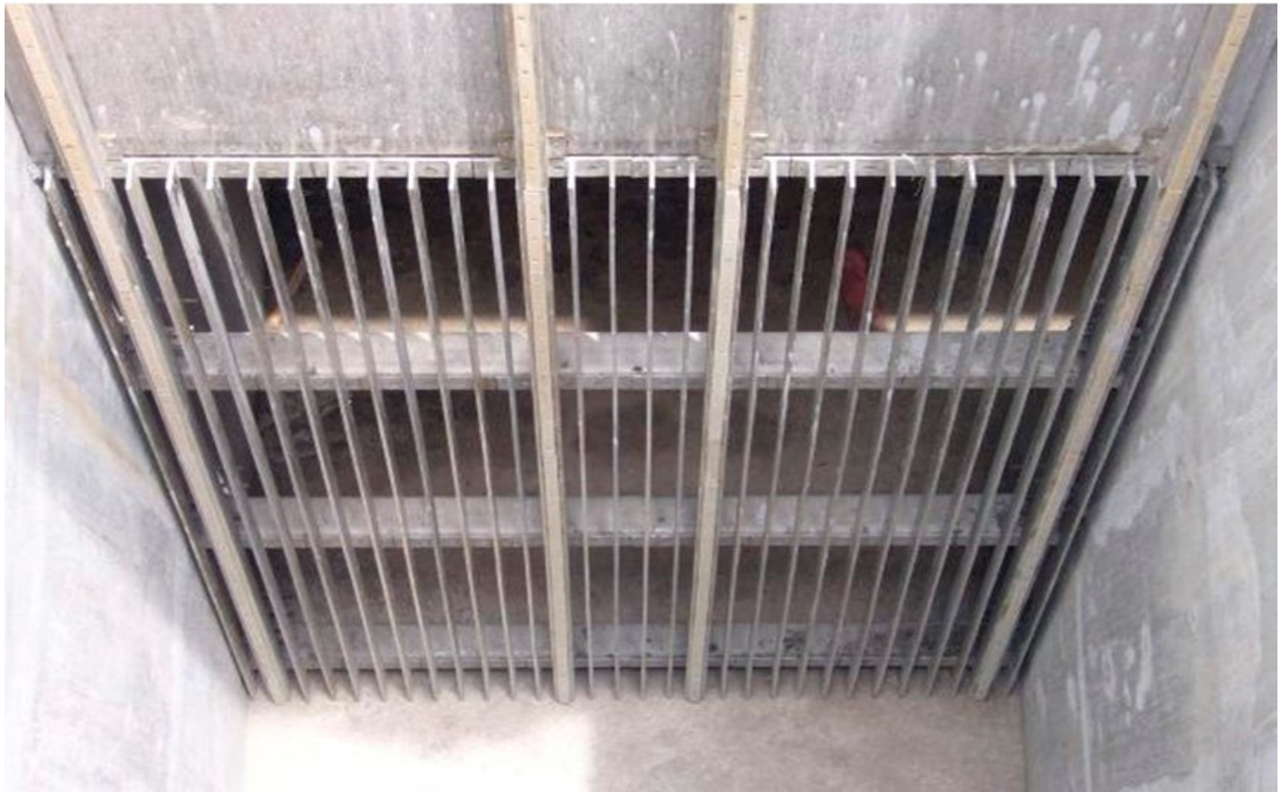
Figure. Four: General Arrangement for Bar Screen.
