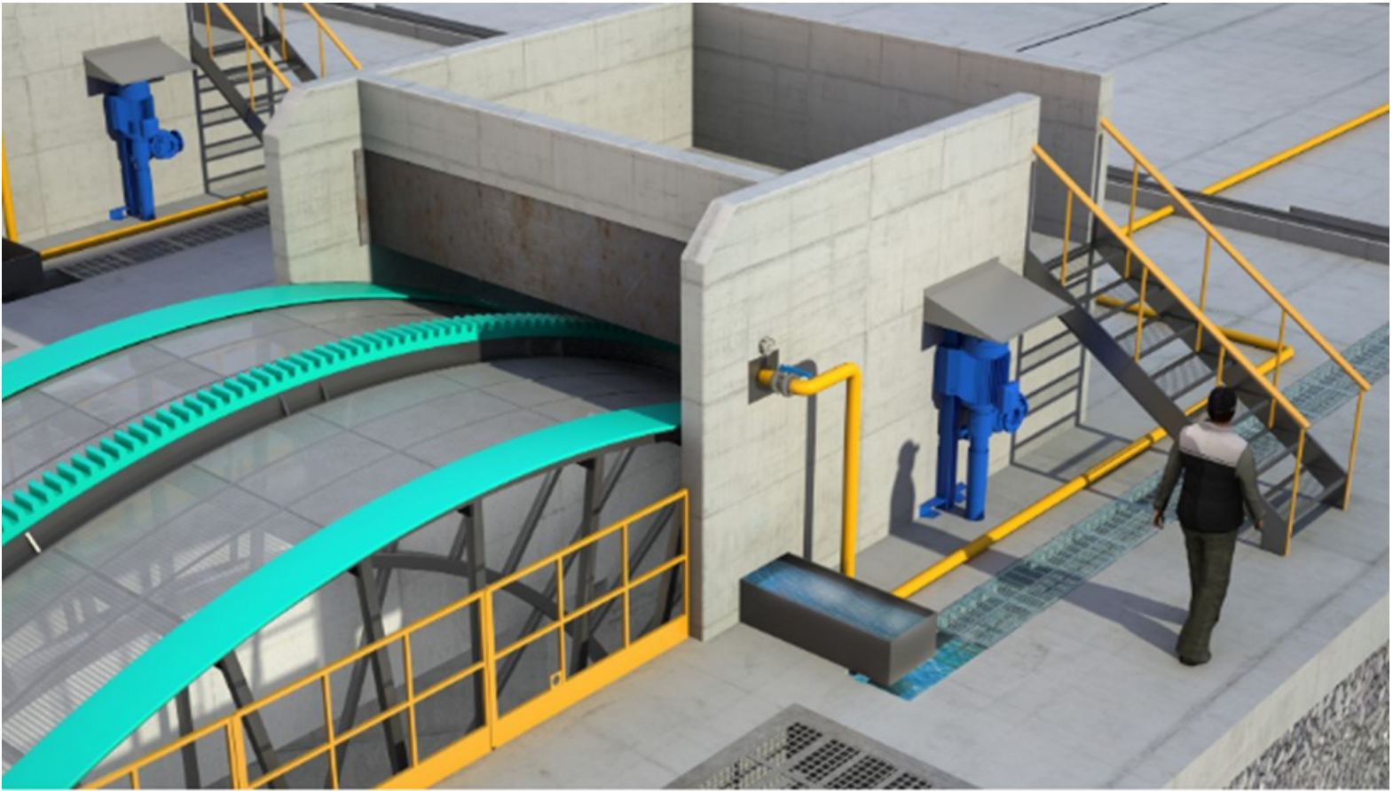
Figure. Ten: Traveling Water Drum Screen type.
