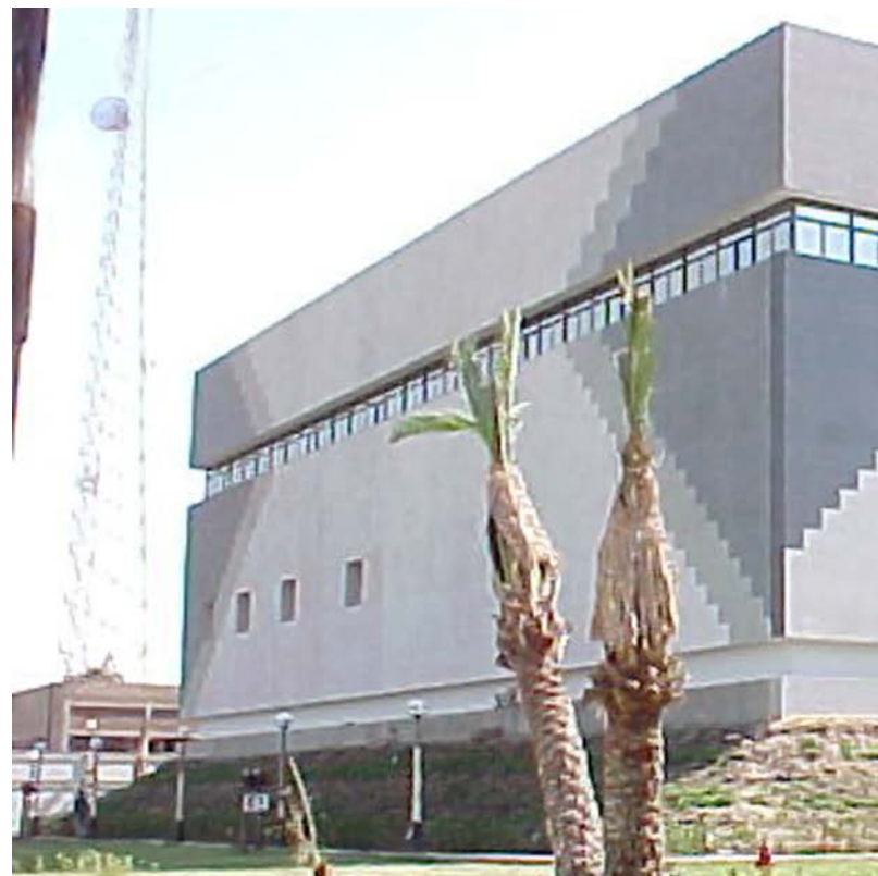
Fig. 7 Cairo Control Center
